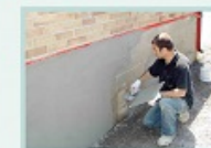
EXTERIOR WALL PLASTERING
