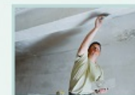
CEILING PLASTERING
