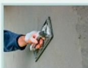
INTERIOR WALL PLASTERING
